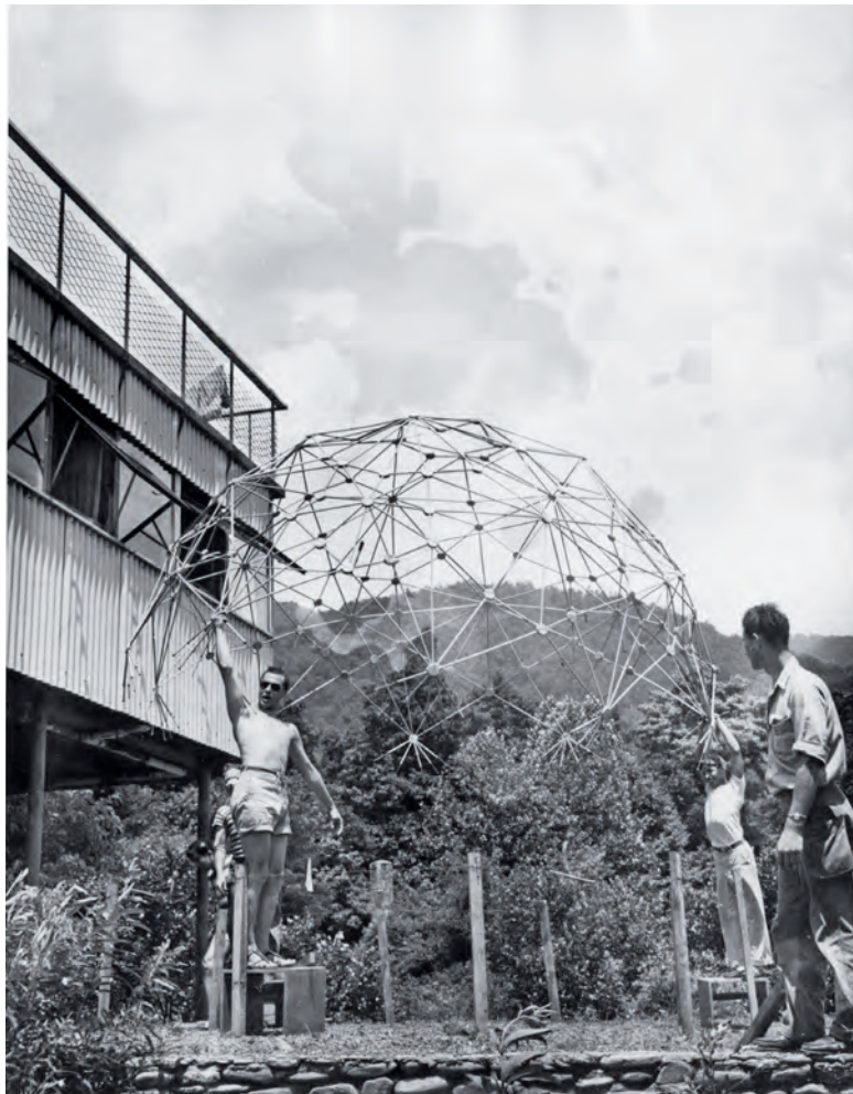
R. Buckminster Fuller's dome assembly at Black Mountain College, 1949 (photograph by Masato Nakagawa; © and provided by State Archives of North Carolina, North Carolina Department of Cultural Resources)
