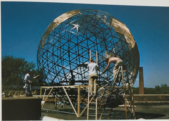
Fig. 28 Students assembling the Geoscope, Cornell University Geodesic Structure 1952
